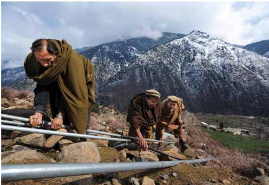
Local IRC workers installing a new water system to replace one destroyed by flooding in the Upper Swat Valley.
